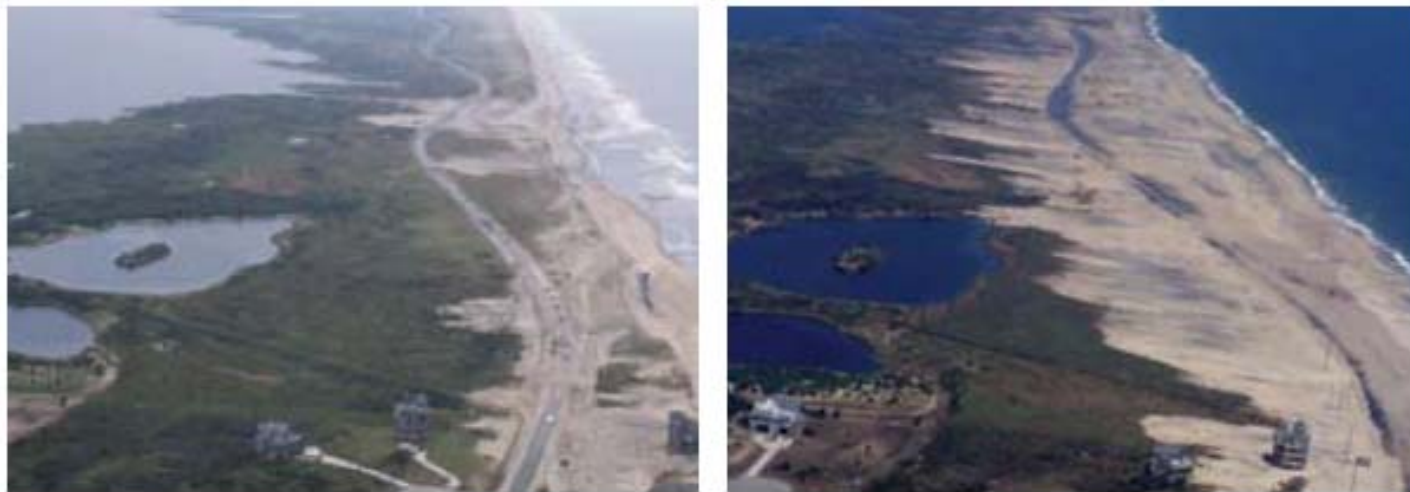
Rodanthe, North Carolina after Hurricane Isabelle, Sept. 2003
